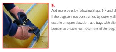
Add more bags by following Steps 1-7 and clip them together. If the bags are not constrained by outer walls and are being used in an open situation, use bags with clips both top and
