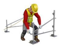
2. Adjust height of frame so that top handrail height will be 1.00m high. Use spirit level to ensure that bottom rail of frame is level. Tighten frame bolts with 7/16th scaffolding spanner.
