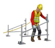
1. Layout equipment and position a pair of Generation Safeguard frames at 3m centres.
